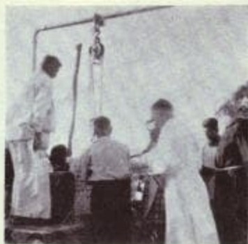
The Principal, Chaplain and Contractors at the foundation stone
