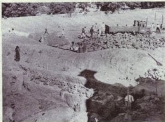
The work begins
