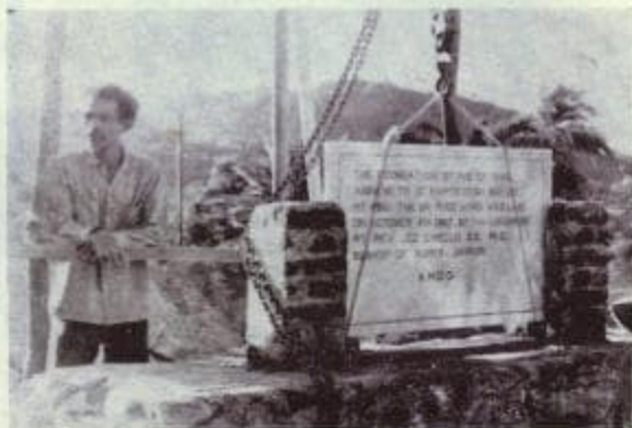
The foundation stone laid
